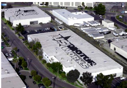
US Motor Works Headquarters, 100,000 sq. ft.
